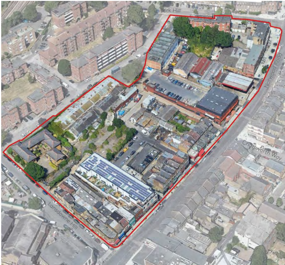
Figure 2 - Site overview image from the south.
