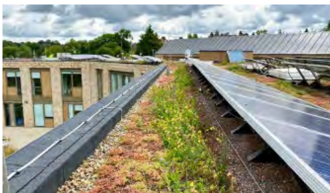
Above left: Biosolar roof at The Ark, Noah's Ark Children's Hospice in London. London Borough of Barnet application 16/5151. Above right: Green roof over bike shed in Hove provides habitat for wildlife, helps to insulate and make buildings more attractive.
