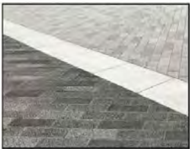
Granolithic block paving Colour: Light/Dark mix with pavement banding [To public realm landscape]
